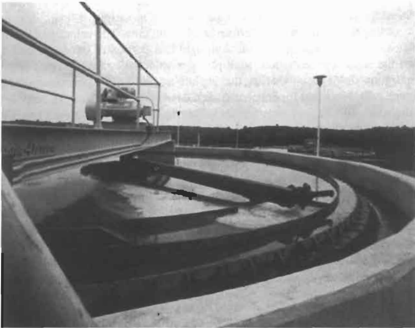
Figure 10-6. Gravity thickener. (Photo courtesy of Dorr Oliver Inc.)
