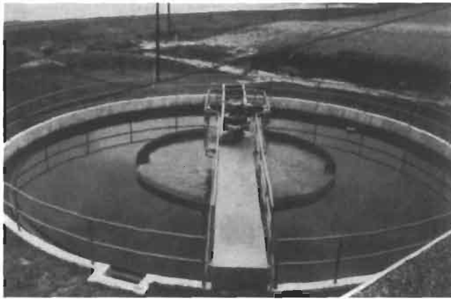
Figure 9-7. Circular settling tank.
