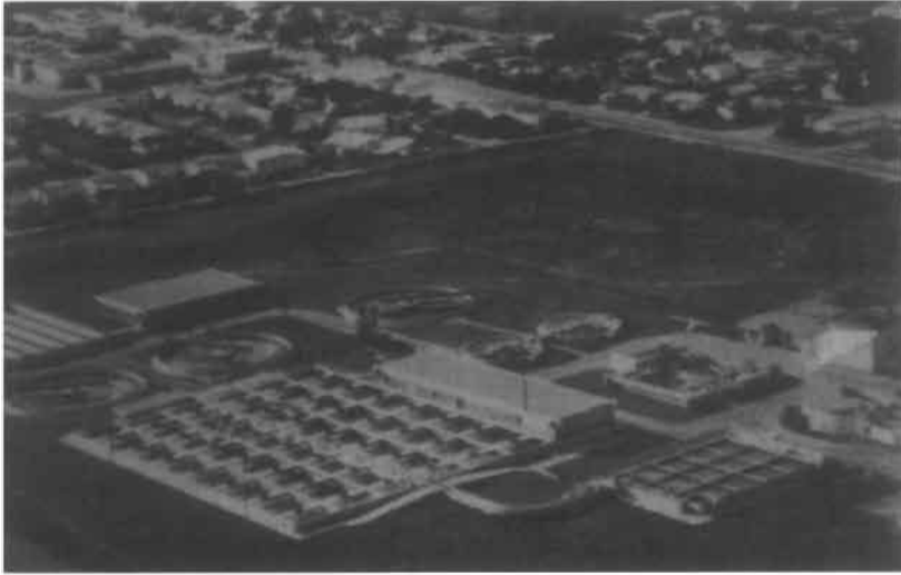
Figure 9-22. An aerial view of a secondary wastewater treatment plant. (Courtesy of Envirex.)
