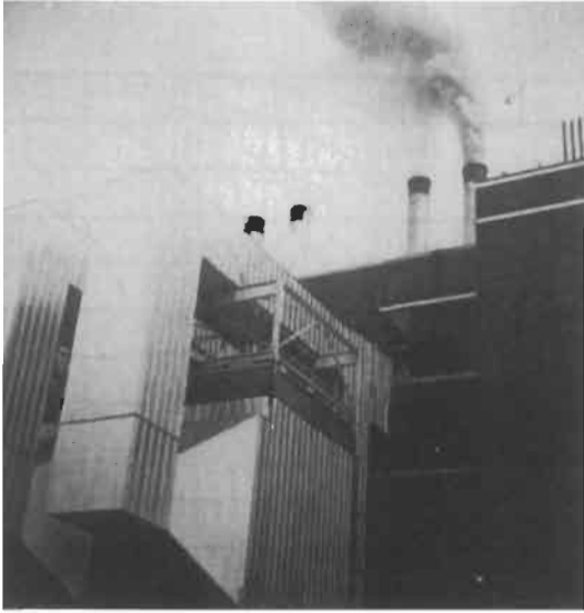
Figure 20-11. Effectiveness of electrostatic precipitators on a coal-fired electric generating plant. The electrostatic precipitator on the right has been turned off.
